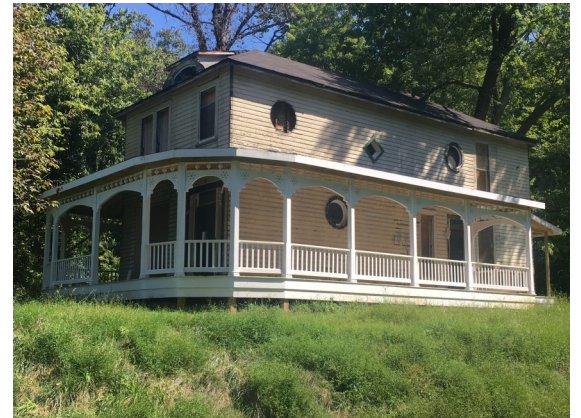
Fully restored porch on the Merriwether House
